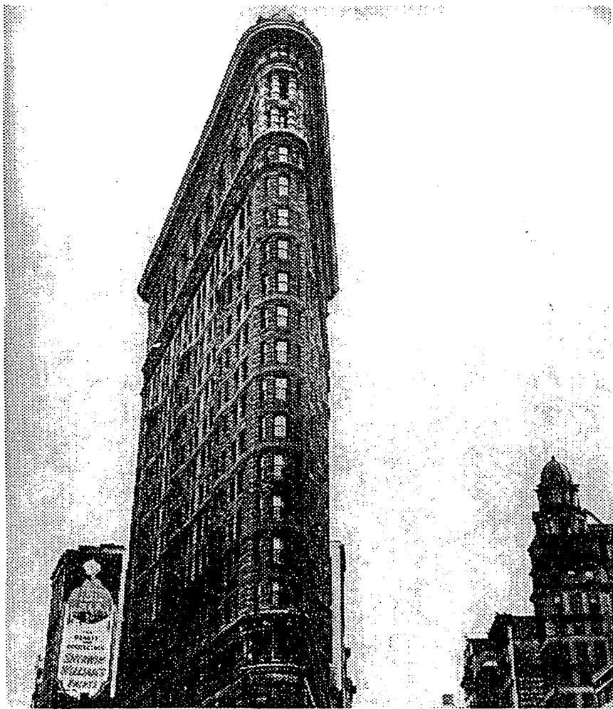
Berenice Abbott's 1938 photo of Flatiron Building, Broadway and 23d Street.
